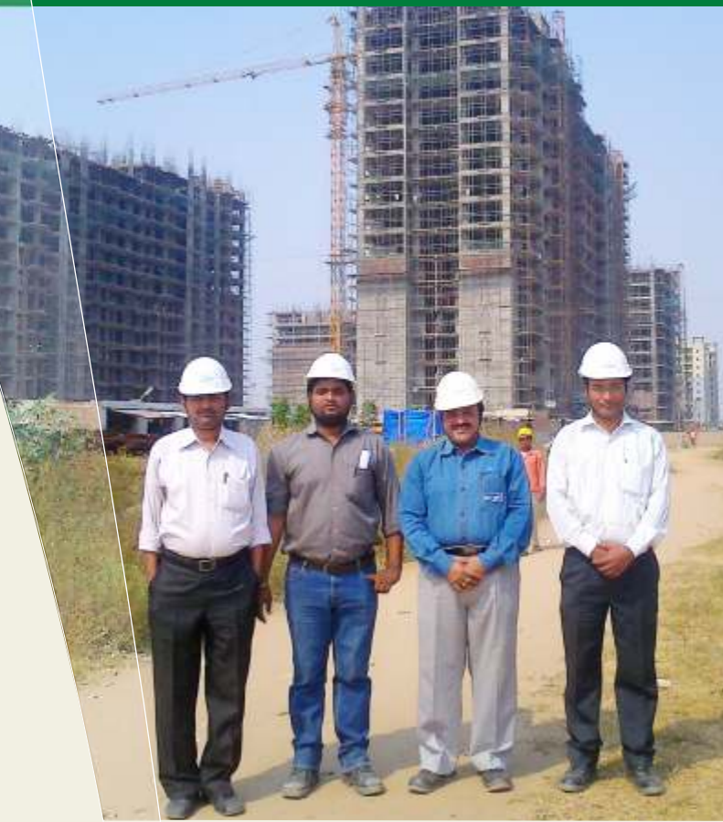
Site office staff at Gurgaon Project location
